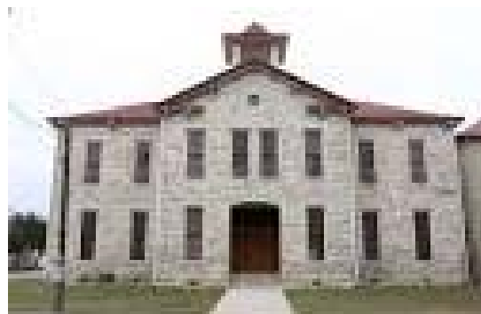
The Navarro building originally opened in 1886 as an elementary school. Today it serves as an academy for grades 9 th through 12 th .
